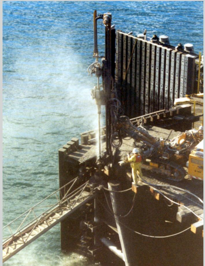
The work was accomplished by craning NWC's drill rig onto a platform at the top of the can, 20' above the water. Service equipment and materials were based on barges surrounding the can.
